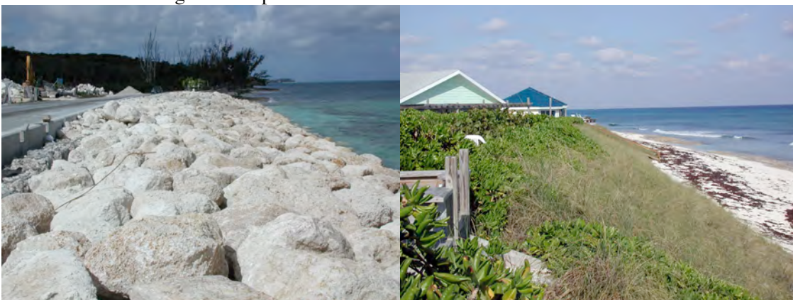
Revetment along West Bay Street, NP.
