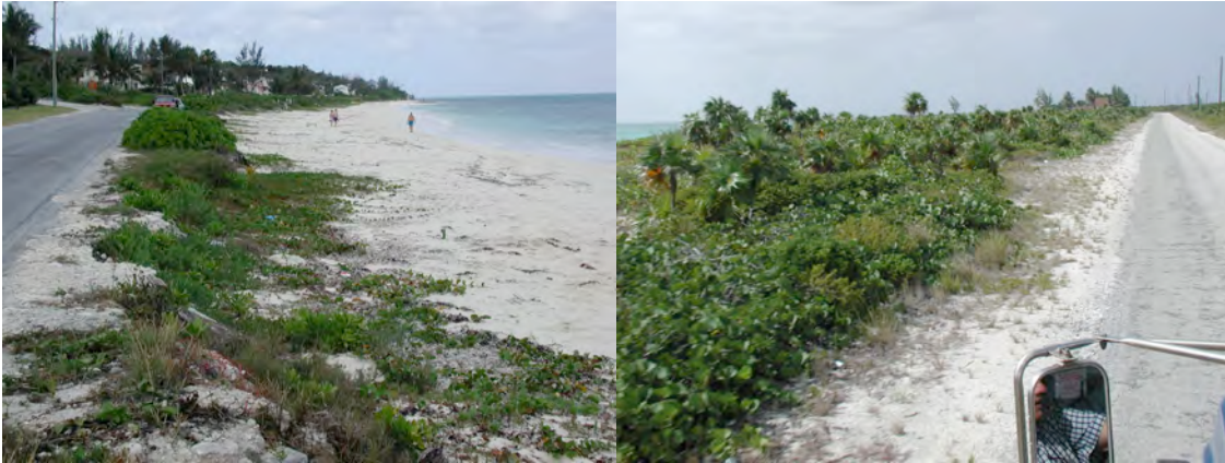
Deteriorated sand dune at Orange Hill, NP Road safely behind dune on San Salvador
