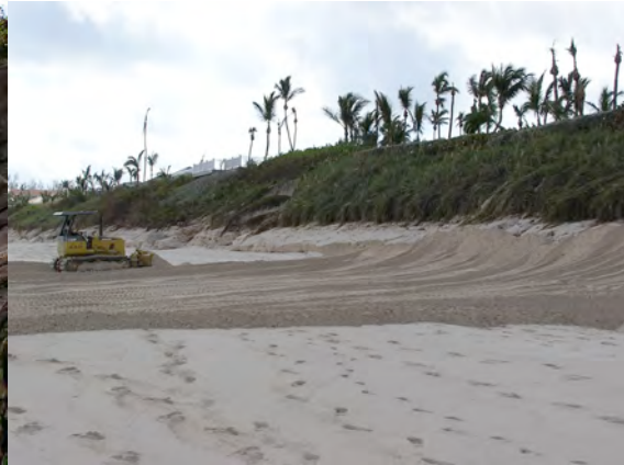
Scraping sand back to dune after H Frances, Paradise Island.
