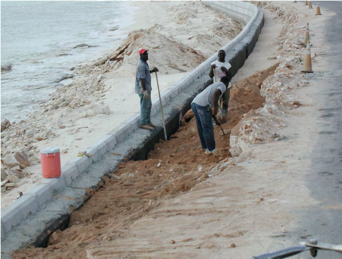
Work on a sea wall on San Salvador
